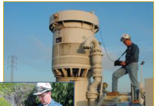
IndustryUptime founder George Dierssen tests a vertical pump (top) and takes performance measurements (left).
